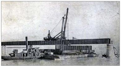
Figure 11. Tug and barge during construction of Knight's Key bridge. (Courtesy of State Library and Archives of Florida, Florida Photographic Collection)
